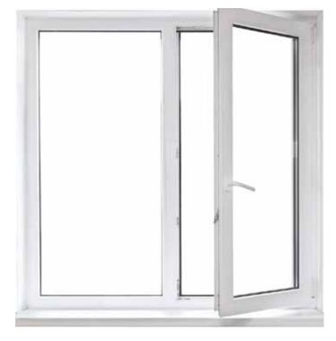
Hinged windows are the most standard kind of windows which are hinged either onto the left or the right side of the windows jamb. This allows them to open inward or out-ward (but not both ways) These windows are manufactured either as a single window, or as a double window.
